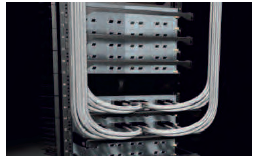
MRJ21 rear cabling
